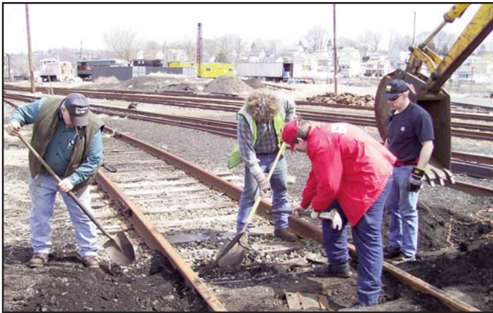
On April 14 th Bob Pitcher, Ira Pollack, James Powell, and Jeremy Rice were digging around a tie as preparation for its being pulled out.
