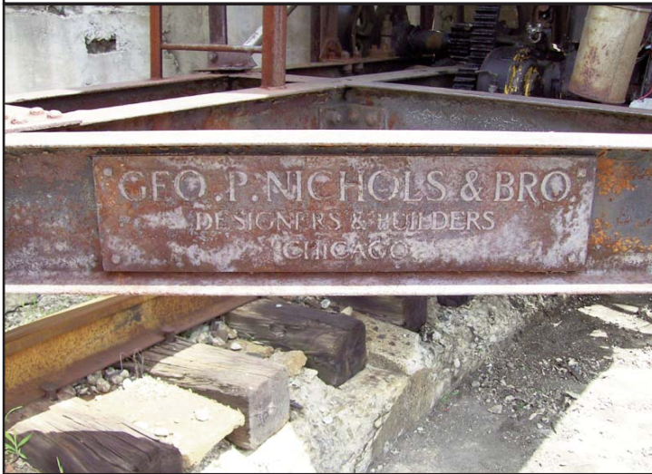
Saulo Araujo and Ed Holowinko scrape rust off the turntable in preparation for rust converter and painting. Below, the manufacturer's plate reads "Geo. P. Nichols & Bro. Designers & Builders Chicago".
