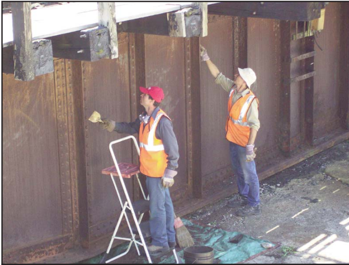
Saulo Araujo and Ed Holowinko scrape rust off the turntable in preparation for rust converter and painting. Below, the manufacturer's plate reads "Geo. P. Nichols & Bro. Designers & Builders Chicago".
