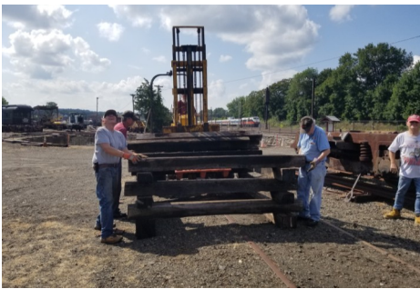
Above: With Secretary Don Konen at the wheel of the forklift, our volunteers construct the cribbing necessary to support the arch when removed from the turntable. Special thanks to Tom McCollough, John Barton, Franz Geren-cir, Don Konen, and Jim Teer for their hard work!
