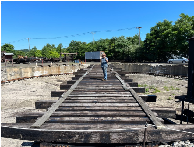
Left: Philip Beard standing on the fully retimbered turntable.
