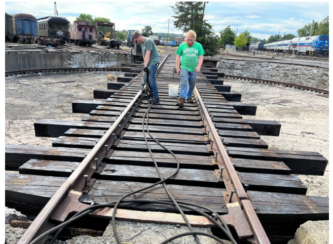
Left: Philip Beard standing on the fully retimbered turntable.
